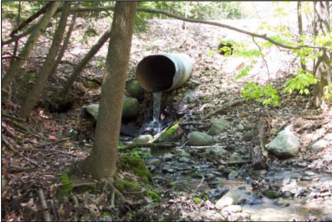
Photo 2.2-2 Another two-culvert design. Severe embedddness has resulted in reduced flow and passage.
