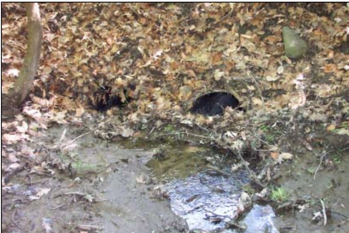
Photo 2.2-2 Another two-culvert design. Severe embedddness has resulted in reduced flow and passage.
